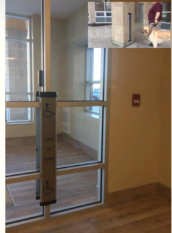
Proper spacing between pulls and door buttons for service dogs
