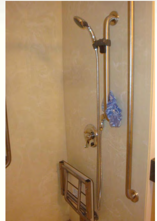
Standard bathroom with folding seat and grab bars
