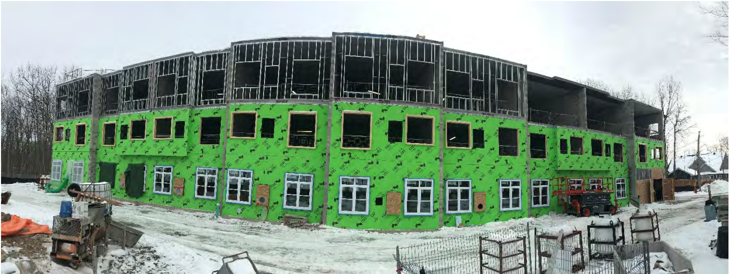
Third Floor Heavy Gauge Steel Framing – West Side
