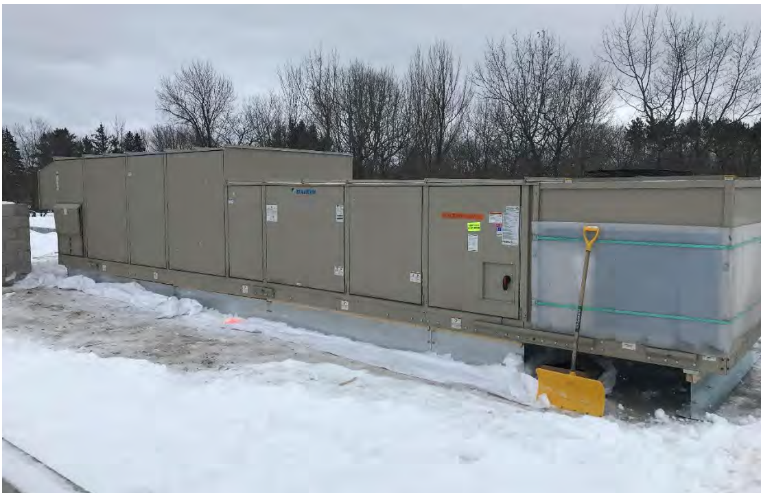
ERV Unit in Place on Flat Roof
