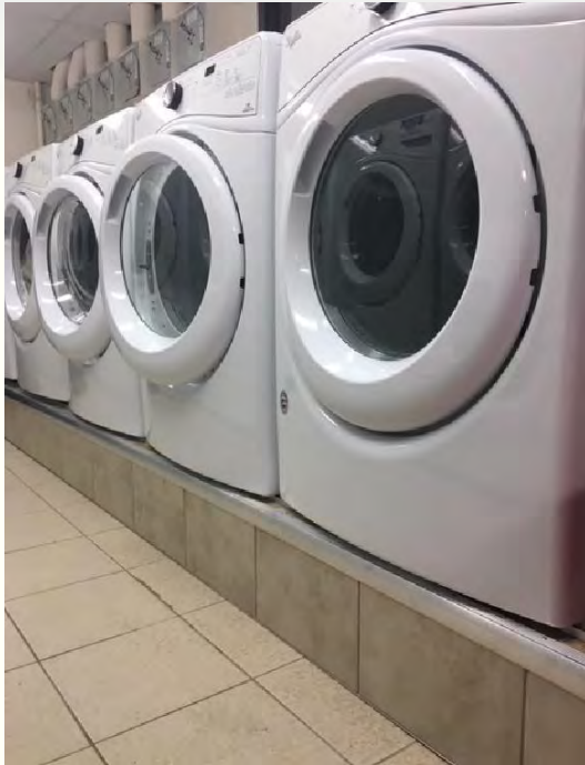
Custom laundry pedestals for optimum working height (200mm)
