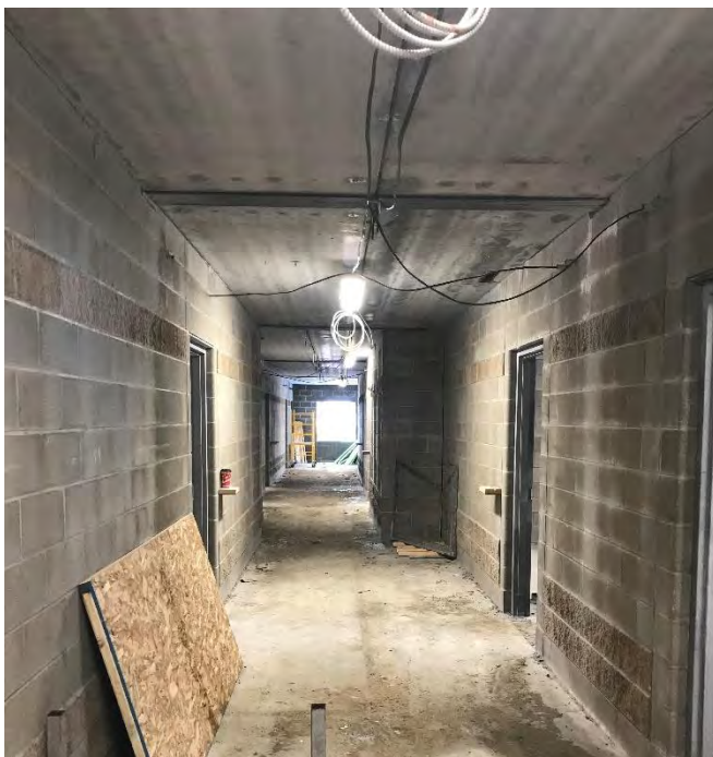
2 nd Floor Temporary Lighting in Corridor
